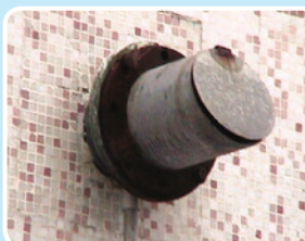
✓ Overflow Pipe with Self-closing Lid
