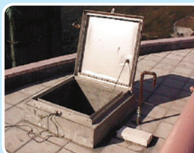
✓ Water Tank with Raised Neck & Double-sealed Cover
