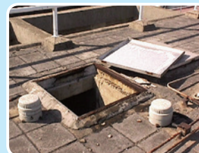
✗ Defective Water Tank Cover
