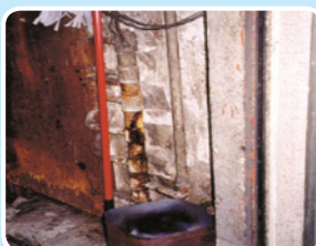
✗ Corroded Water Pipe
