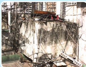
✗ Poorly Maintained Water Tank
