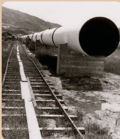
A large pipeline with a diameter of 48 inches was laid in 1960 for the reception of water from the Shenzhen Reservoir.
