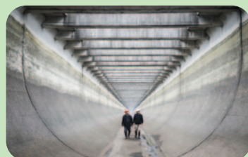
Inside view of the closed aqueduct at Jinhu during water suspension for maintenance
