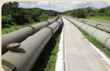
Water pipelines in Hong Kong for conveying Dongjiang water
