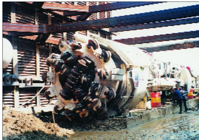
建造輸水隧道用的巨型隧道鑽挖機。 Giant tunnel boring machine for the construction of the inlet tunnel.
