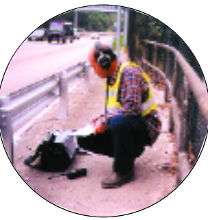
以最先進的儀器進行地下喉管測漏工作。 Using state-of-the-art equipment to detect underground pipe leaks.
