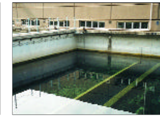
北港濾水廠的濾水池。 Filter in Pak Kong Treatment Works.
