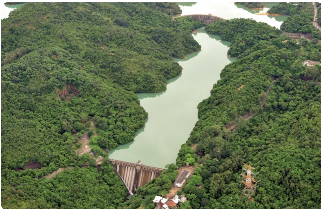
透過水塘間轉運計劃，九龍副水塘的溢流得以輸送到沙田濾水廠。 The flood water from Kowloon Byewash Reservoir is carried to Sha Tin Water Treatment Works through an Inter-reservoirs Transfer Scheme.
