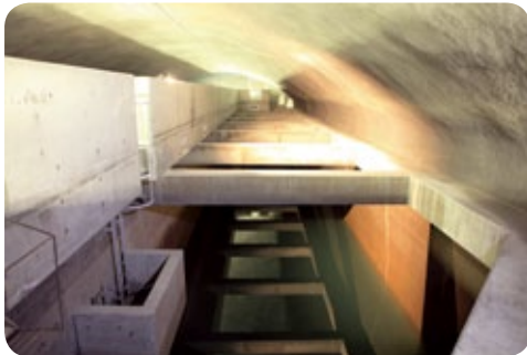
善用土地資源，把西區海水配水庫重置於石洞中。 Salt water service reservoirs are constructed inside a rock cavern to optimise land use.
