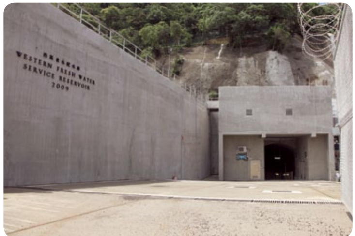
善用土地資源，把西區海水配水庫重置於石洞中。 Salt water service reservoirs are constructed inside a rock cavern to optimise land use.
