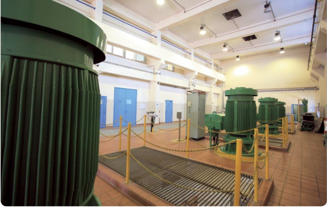
從海中抽取的鹹水，在海傍海水抽水站經過濾隔及消毒後成為沖廁用水。 Salt water, extracted from the sea, becomes flushing water after screening and disinfection at a seafront salt water pumping station.
