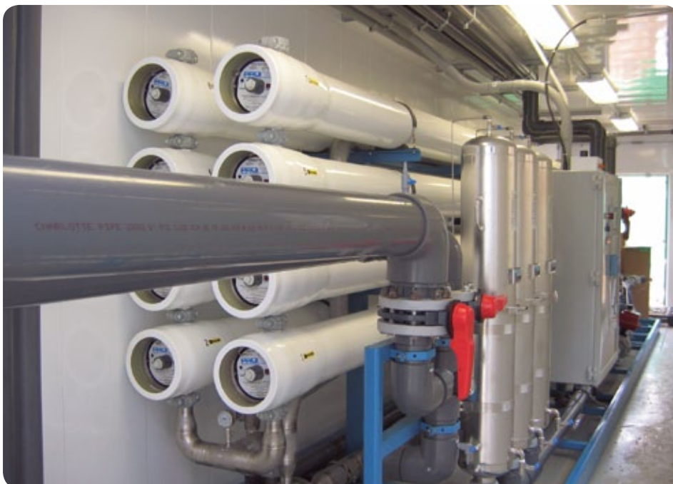
以逆滲透技術在香港進行海水淡化，技術上是可行的。 Using reverse osmosis technology for sea water desalination is technically viable in Hong Kong conditions.
