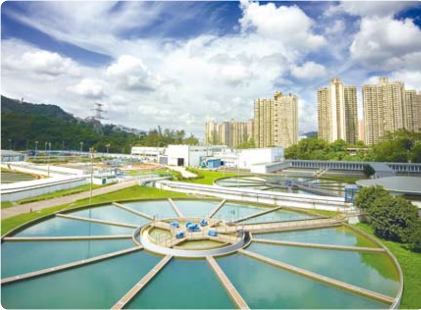
於一九六四年落成的沙田濾水廠是本港目前投產量最高的濾水廠。 Commissioned in 1964, Sha Tin Water Treatment Works is currently the largest in Hong Kong in terms of production capacity.
