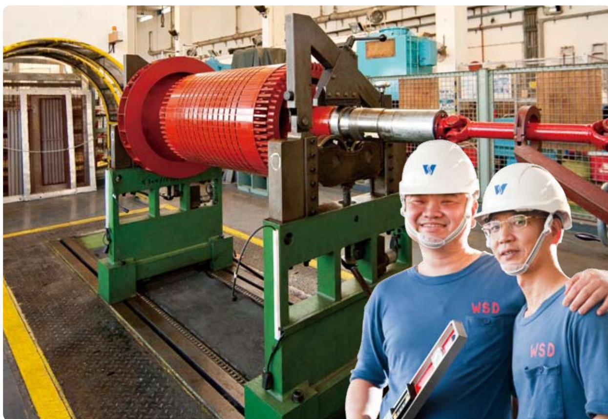
一水泵的電動機在維修中。 An electric pump motor being maintained.
