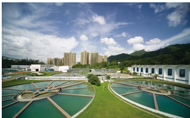
(上) 掘路工作在進行中。 (upper) Road opening work in progress. (下) 沙田濾水廠 (lower) Sha Tin Water Treatment Works.
