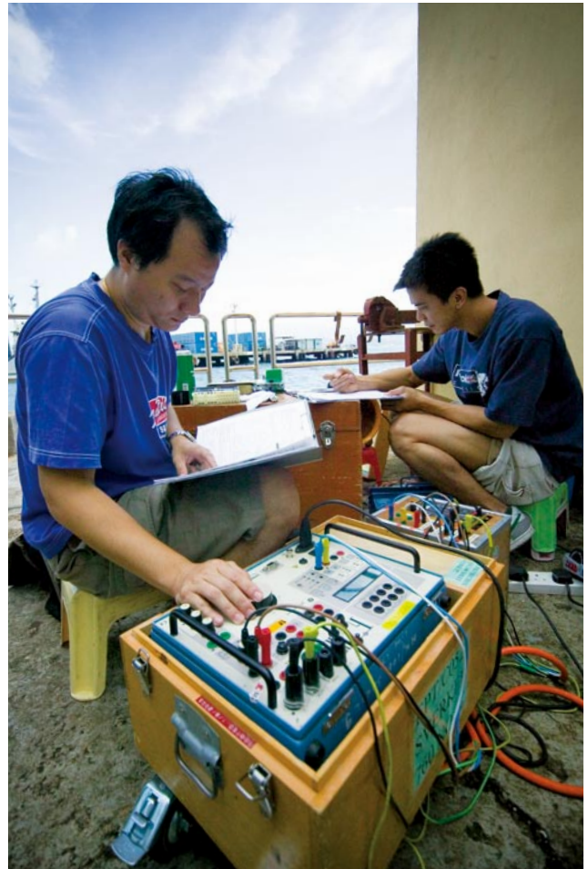
對設備進行測試。 Staff performing test on plant equipment.
