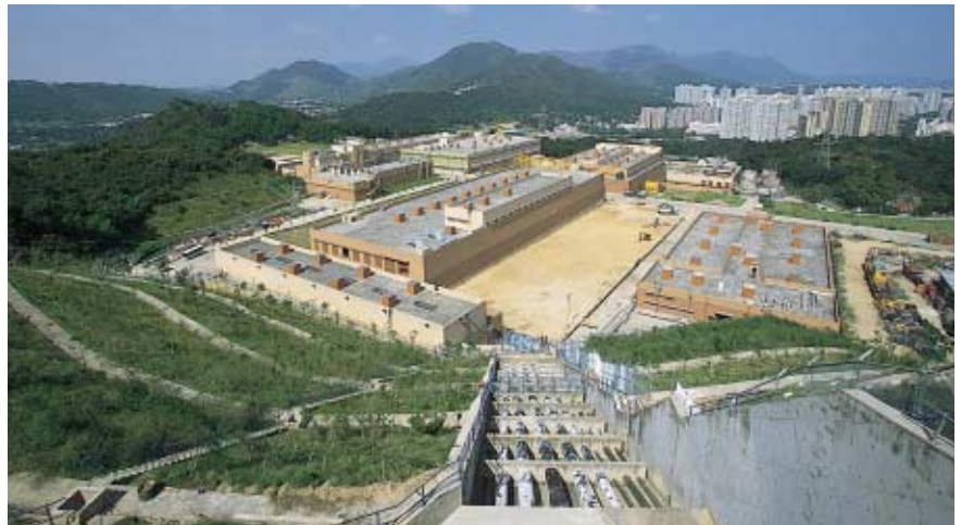
將近落成的大埔濾水廠。 Nearly completed Tai Po Water Treatment Works.
