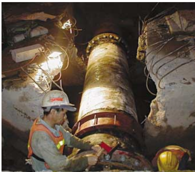
員工正搶修一條爆裂水管。 A burst water main being repaired.
