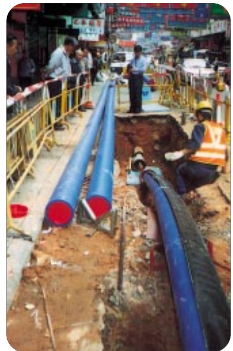
敷設聚乙烯管。 Polyethylene pipes being laid.
