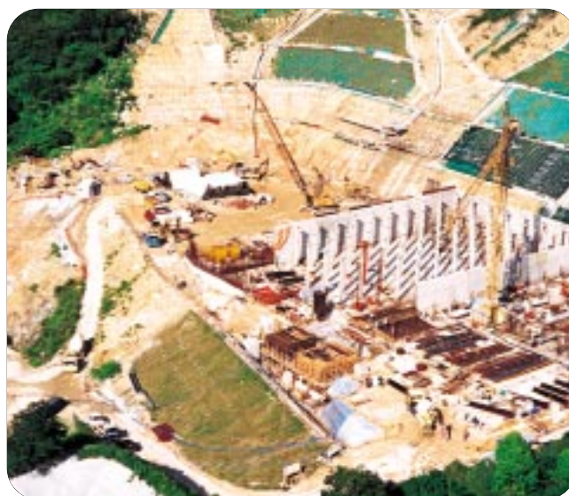
興建中的食水配水庫。 Fresh water service reservoir under construction.
