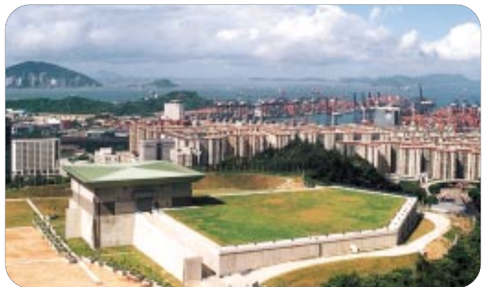
蝴蝶谷食水主配水庫。 Butterfly Valley Fresh Water Primary Service Reservoir.
