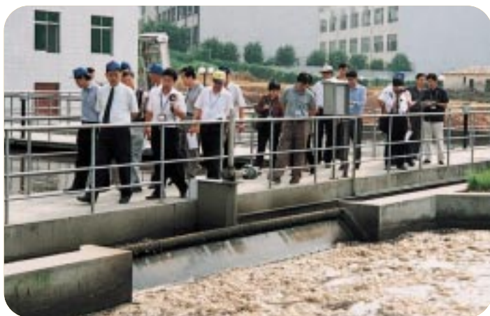
水質事務諮詢委員會代表團參觀位於廣東的污水處理廠。 Delegation of the Advisory Committee on the Quality of Water Supplies visiting a wastewater treatment works in Guangdong.
