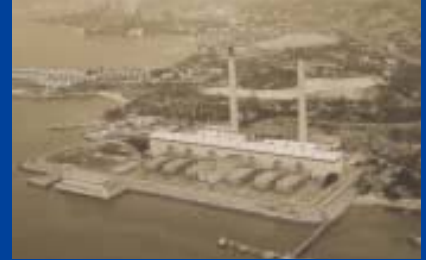
樂安排海水化淡廠 Lok On Pai Desalting Plant
