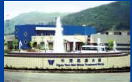
使用臭氧及生物濾池的牛潭尾濾水廠 Ngau Tam Mei Water Treatment Works using ozone and biological filters
