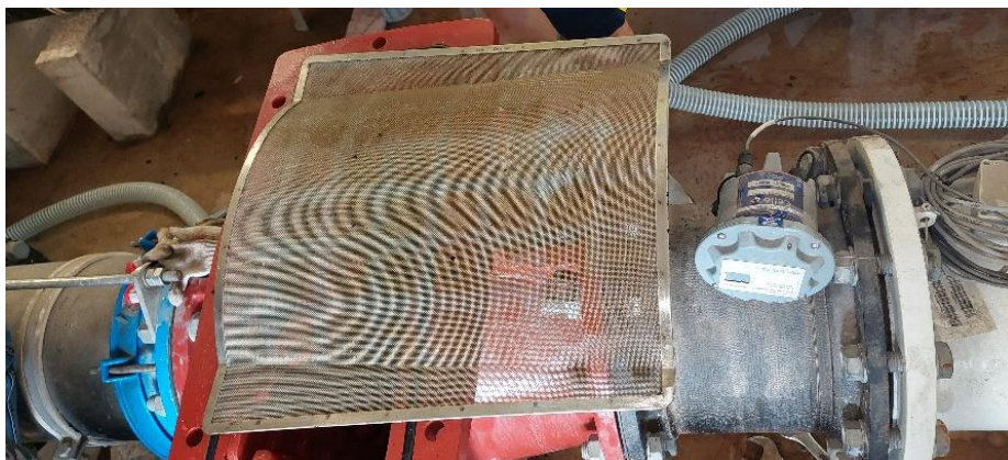
Photo 6 – Take out the screen for flushing
