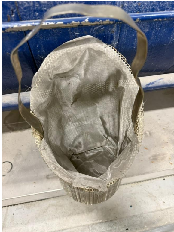
Photo 3 – Take out the screen for flushing
