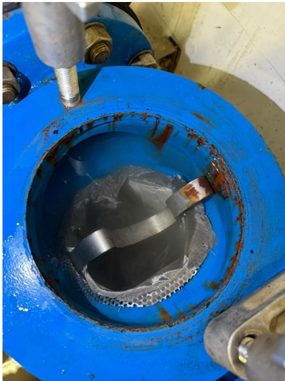
Photo 2 – Open the removal Cap of the strainer
