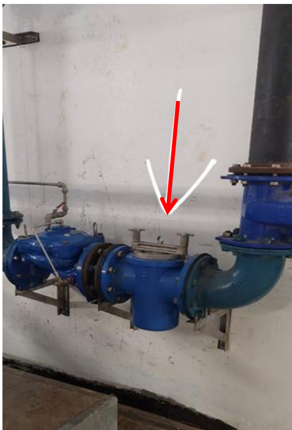
Photo 1 & 1A – Strainer near check meter position of the communal service to individual building block
