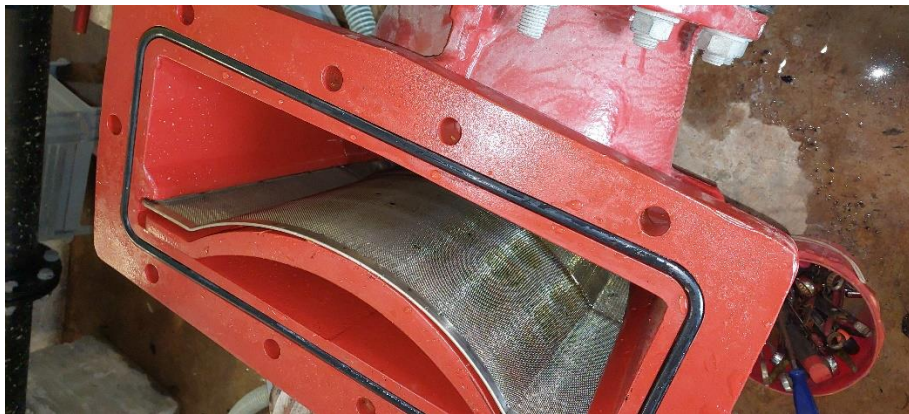
Photo 5 – Open the removal cap of the filter
