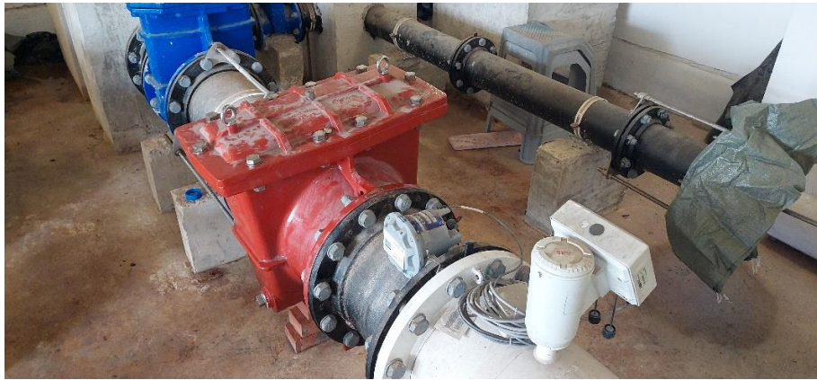
Photo 4 – Filter before sump tank
