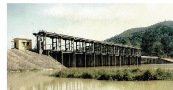
Works including extension of water supply canals, channels and pumping stations.
