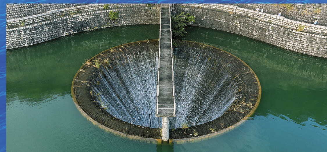
Bellmouth Overflow at Shing Mun Reservoir
