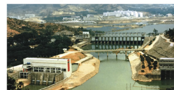
Works including upgrading of pumping stations at Dongjiang, Shima, Matan, Zhutang and Shaling, etc and expansion of artificial channels and natural rivers.
