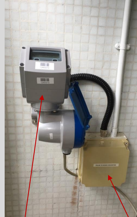
EM water meter converter generating pulse output
