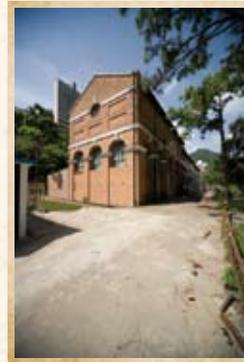
The station's role was to pump water from this southern most part of Hong Kong Island's catchment to the tunnel inlet located at the middle of the hill. Its engine hall is a rare piece of historic industrial architecture. The warehouse styled building, red brick walls and Chinese tiled pitched roofs encase the engine house which, over the decades, has contained steam driven pumps capable of transferring 3 million gallons (14 000 cubic metres) of water per day.
