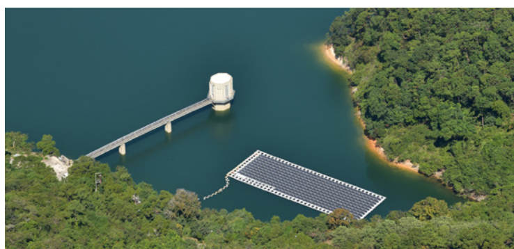
石壁水塘的浮動太陽能板發電系統 Floating PV System at Shek Pik Reservoir
