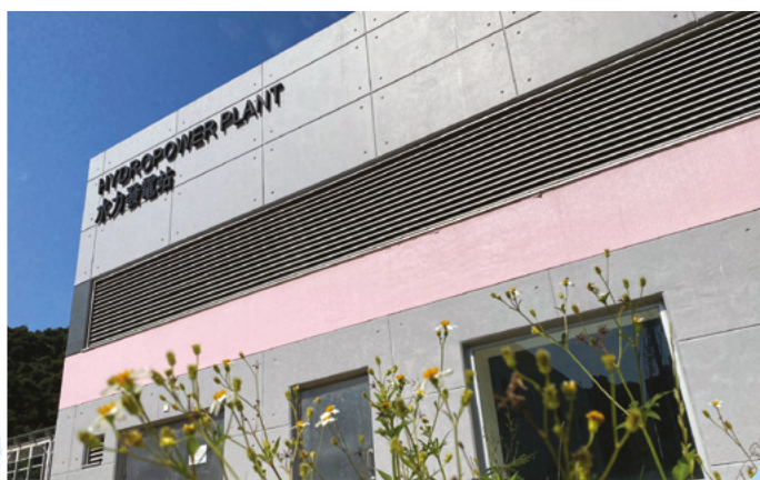
沙田濾水廠的水力發電站 Hydropower Plant at Sha Tin Water Treatment Works
