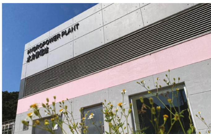
沙田濾水廠的水力發電站 Hydropower Plant at Sha Tin Water Treatment Works
