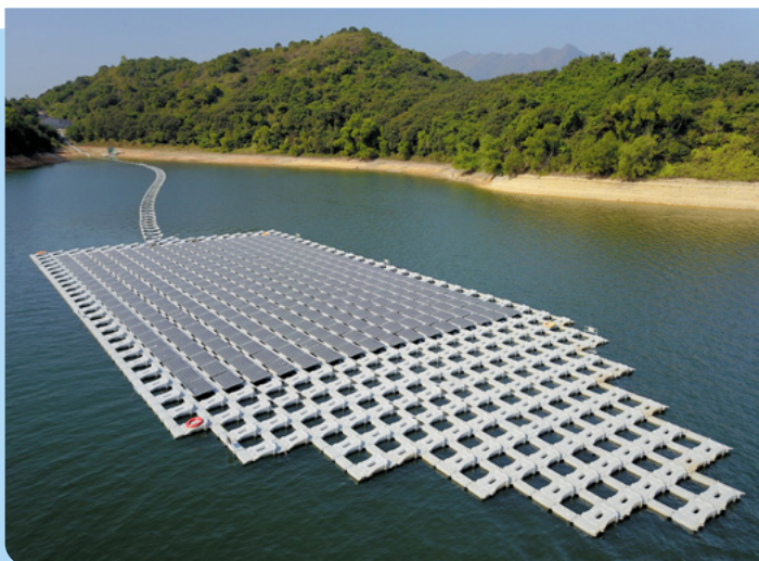
船灣淡水湖的浮動太陽能板發電系統 Floating PV System at Plover Cove Reservoir
