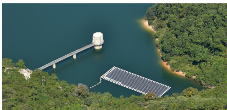
石壁水塘的浮動太陽能板發電系統 Floating PV System at Shek Pik Reservoir
