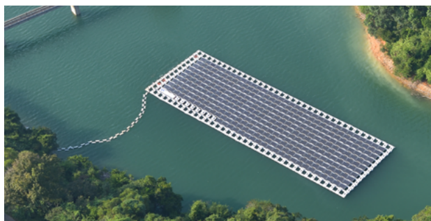
石壁水塘的浮動太陽能板發電系統 Floating PV System at Shek Pik Reservoir
