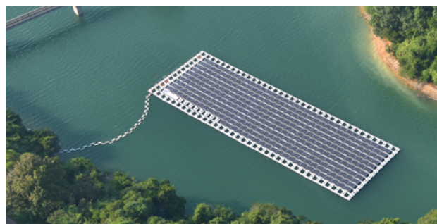
石壁水塘的浮動太陽能板發電系統 Floating PV System at Shek Pik Reservoir
