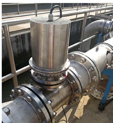
▲ 內聯閉式水力發電裝置 In-line Hydropower Harness Device
