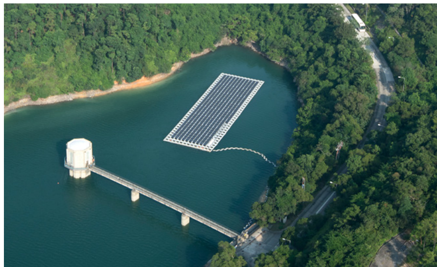
▲ 石壁水塘的浮動太陽能板 Floating PV System at Shek Pik Reservoir
