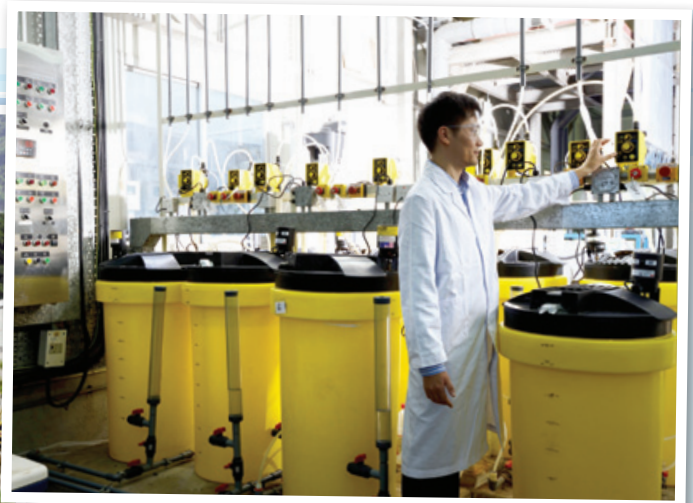
試驗研究廠用作測試擬用於沙田濾水廠南廠的處理工藝流程。 Pilot plant for testing the proposed treatment process for Sha Tin Water Treatment Works – South Works.
