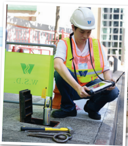
正進行滲漏檢測。 Conducting leak detection tests.
