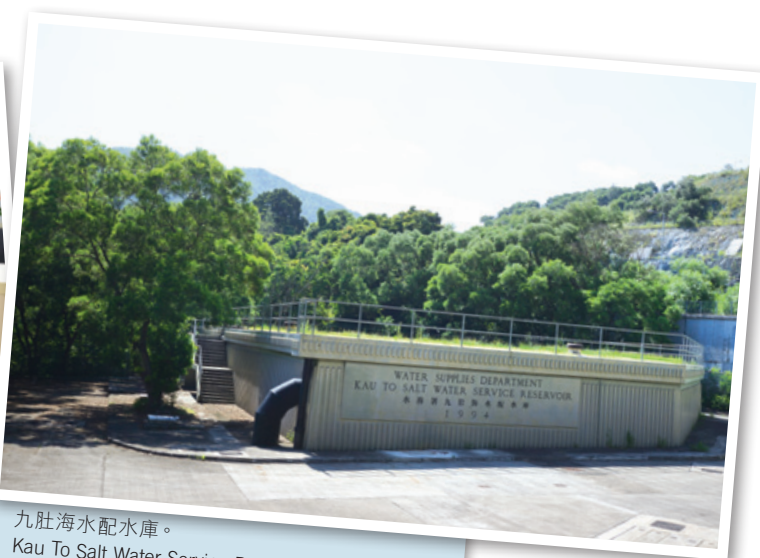
擴建沖廁用的海水供應系統，以節省珍貴食水。 Saving fresh water by extending the sea water supply network for flushing.
