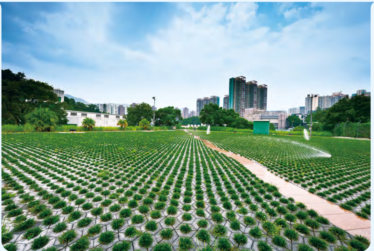
屯門濾水廠內清水池的綠化屋頂。 The green roof of the clear water tank in Tuen Mun Water Treatment Works.
