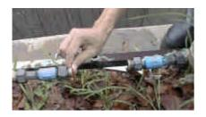
Install the two gaskets on the inlet and outlet of the tail pieces.
