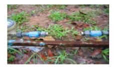
Turn on the valve/stopcock and flush the pipe clean with water. Turn off the valve/stopcock. Install the tail pieces and coupling nuts onto the inlet and outlet of the water pipes, tighten with pipe wrenches. Use Teflon sealing tape as required. Ensure that the distance between the inlet and outlet tail pieces is between 110 to 113 mm.
