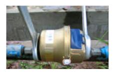
Tighten the nuts with two spanners simultaneously. If the meter rotates and the counter faces wrong direction, rotate the meter back by hand before proceeding to tighten the nuts further.
