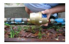
Position the TD88 meter in between the inlet and outlet tail pieces with the counter facing upward. While holding the meter with one hand, install the nuts one at a time onto the meter with the other hand. Ensure that the gaskets do not fall out.
