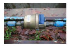
Turn on the valve/stopcock to check for leaks.
