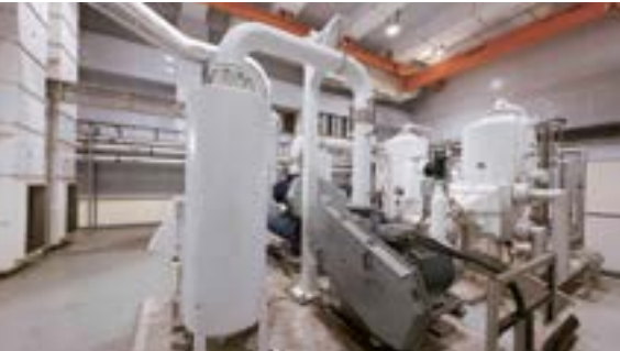
▲ The vacuum pressure swing absorption system at Tai Po Water Treatment Works extracting oxygen from the air.
