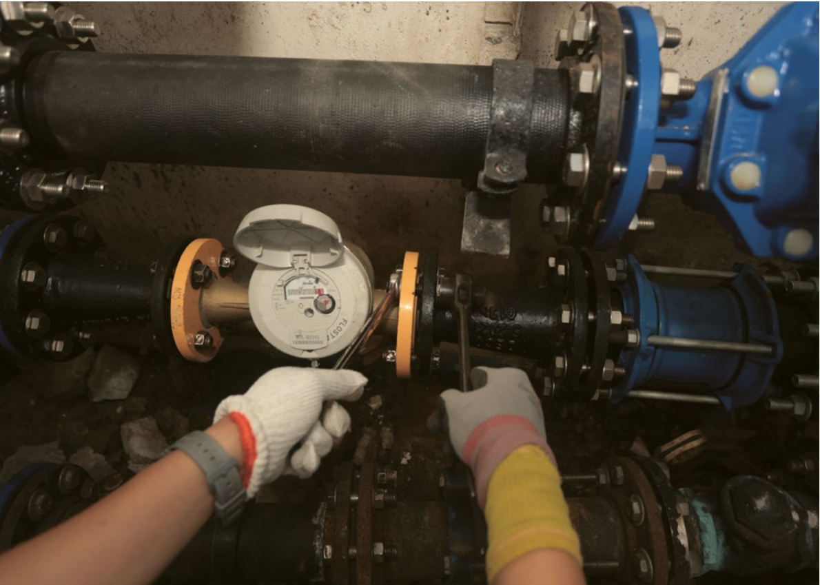
▲ Waterworks staff installing water meter
