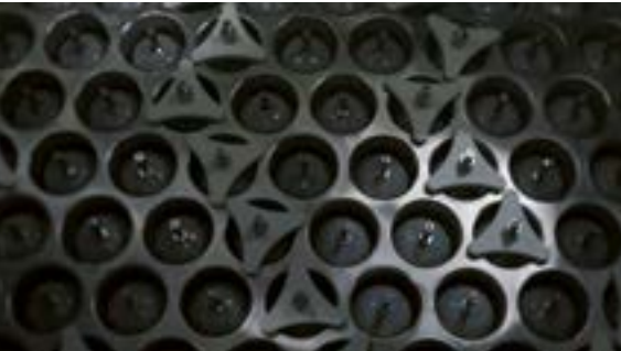
▲ The ozone generator at the Tai Po Water Treatment Works simulates the way ozone is produced in nature by lightning, using high voltage electricity to convert oxygen into oxygen molecules, which are then combined to form ozone.
