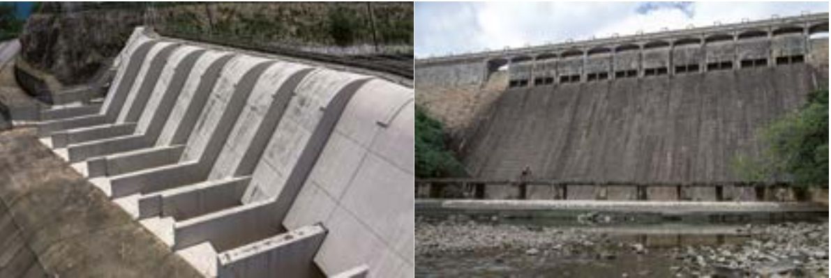
▲ Spillways of the subsidiary dam of Plover Cove Reservoir (left) and Tai Tam Tuk Reservoir dam (right)
