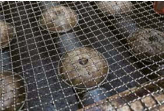
▲ Aerators are installed in the Dongjiang water supply mains. An air-blower is activated to inject a large amount of air to keep water flowing at the bottom of the incoming channel, thus reduce stagnant water areas.
