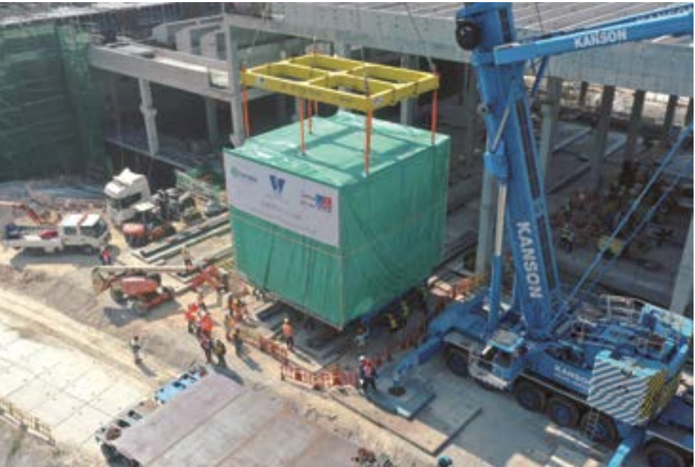
▲ A giant crane lifts the 90-tonne RO racks onto temporary tracks during its installation prior to the completion of the building's structural frame
