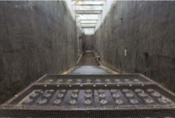
▲ Muk Wu Raw Water Pumping Station during maintenance. The intake culvert is filled with water when in operation.
