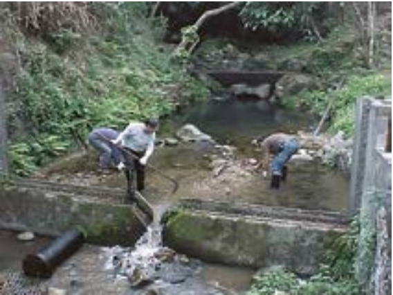
▲ Waterworks staff clearing sediment adjacent the weir
