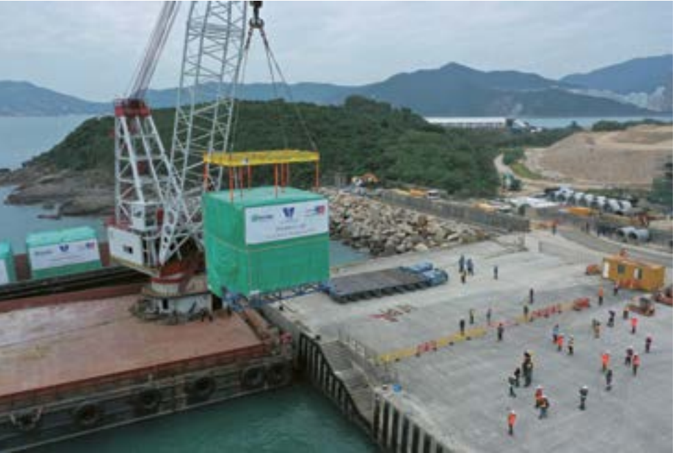
▲ The RO racks arriving at the site of the Tseung Kwan O Desalination Plant
