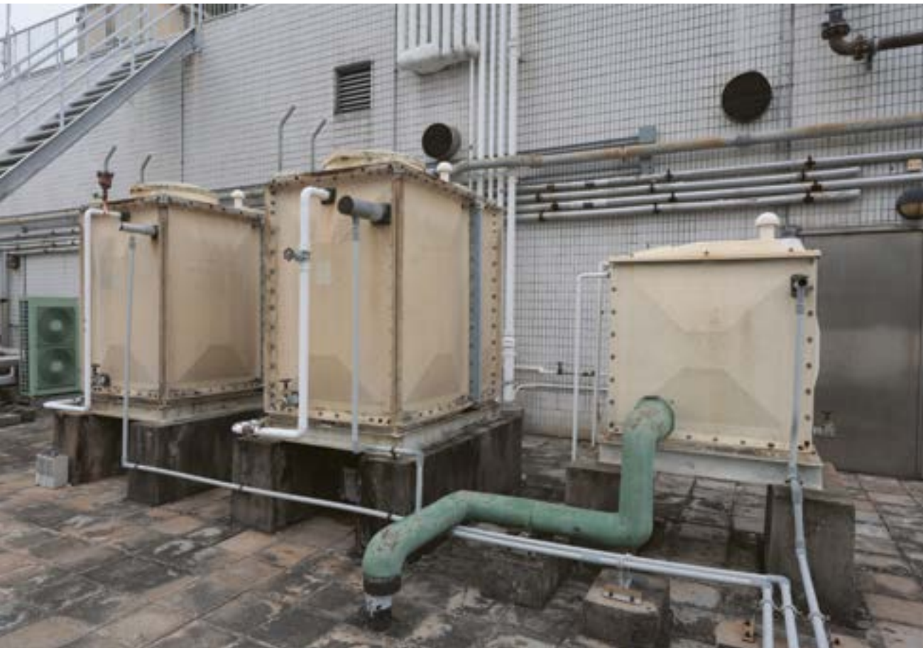
▲ Water storage tanks on the rooftop of a building
