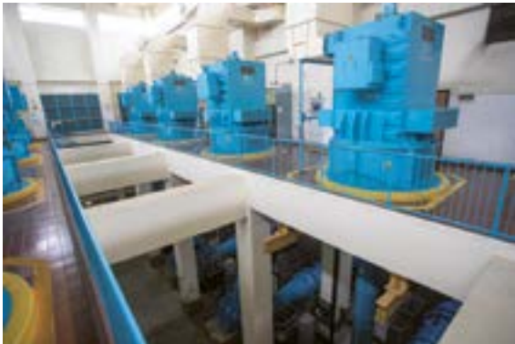
▲ The pump is two-storey high, with the motor on the top driving the impeller of the rotary pump at the bottom to generate a centrifugal force, which drives the rotation of Dongjiang raw water for transportation.
