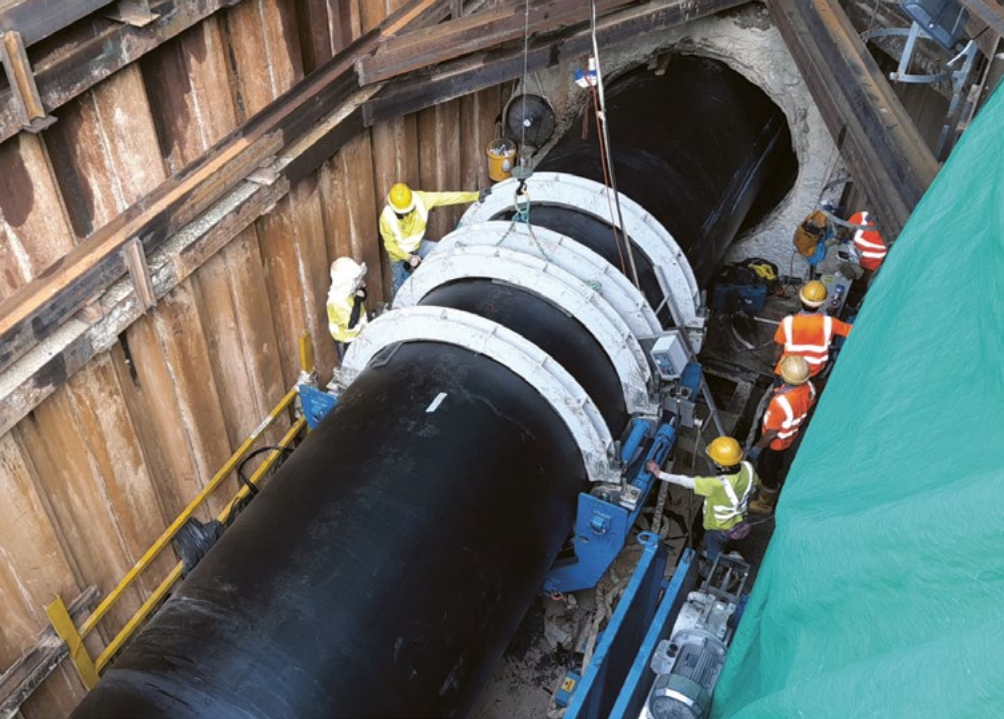
▲ Improvement to Dongjiang water mains P4 - insertion of a reshaped polyethylene pipe into the existing water mains during large-scale rehabilitation work.
