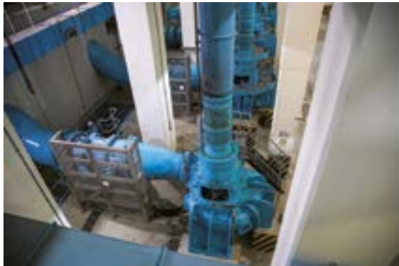
▲ The motor pushes the balance shaft to drive the pump and transfers the raw water to impounding reservoirs or water treatment works.
