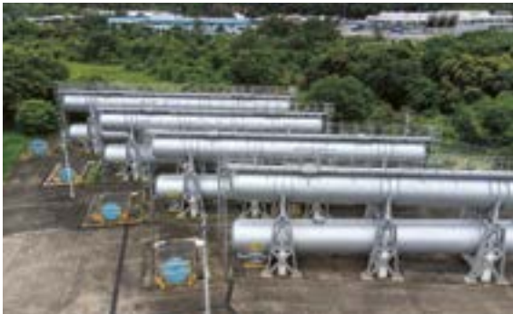
▲ The MWRWPS is equipped with a buffer tank (also known as a surge vessel) connected to the Dongjiang raw water mains, with a 50/50 split between raw water and compressed air. This device is usually located in water mains that have many bends, so as to alleviate the problem of rapid pressure increases caused by water hammering. In the event of a mains burst causing a sudden drop in pressure, the raw water in the surge vessel is replenished to balance the water pressure in the pipe and protect the pump which is constantly running.
