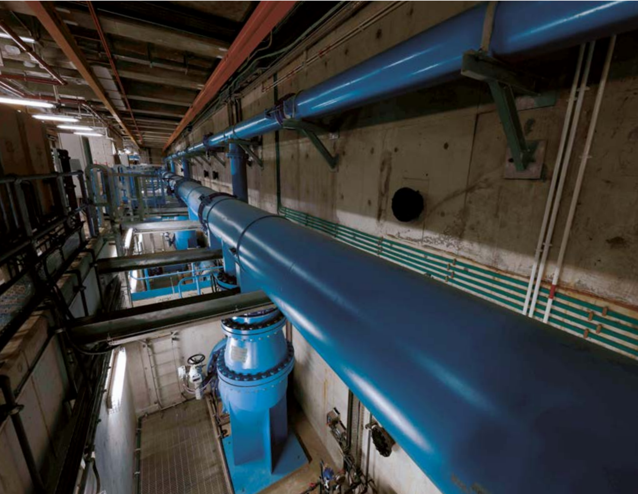
▲ The principal mains of the Water Treatment works
