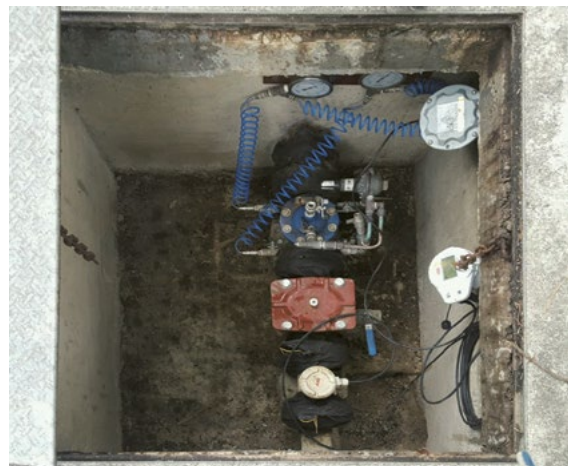
▲ Equipment and device in the District Metering Area chamber
