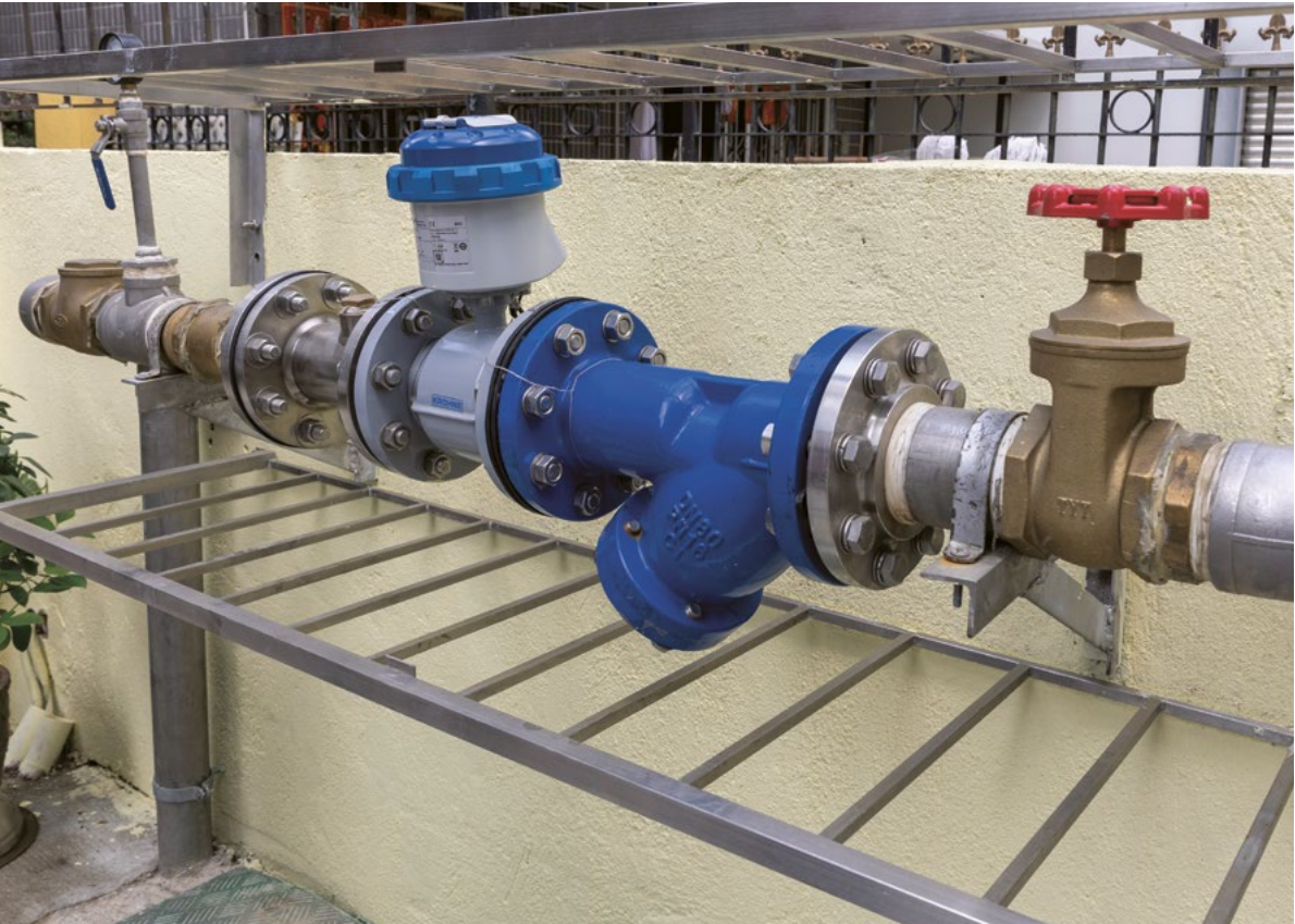
▲ WSD water meters connected to a building's inside service
