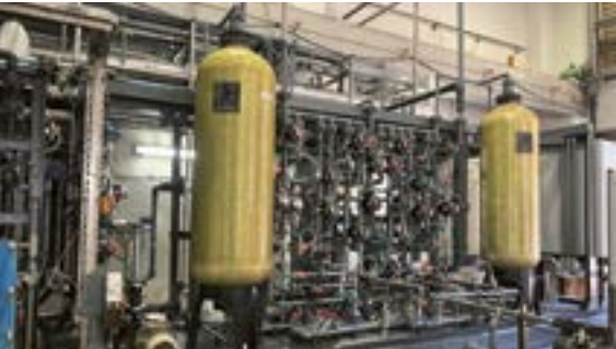
▲ On-site chlorine generation
