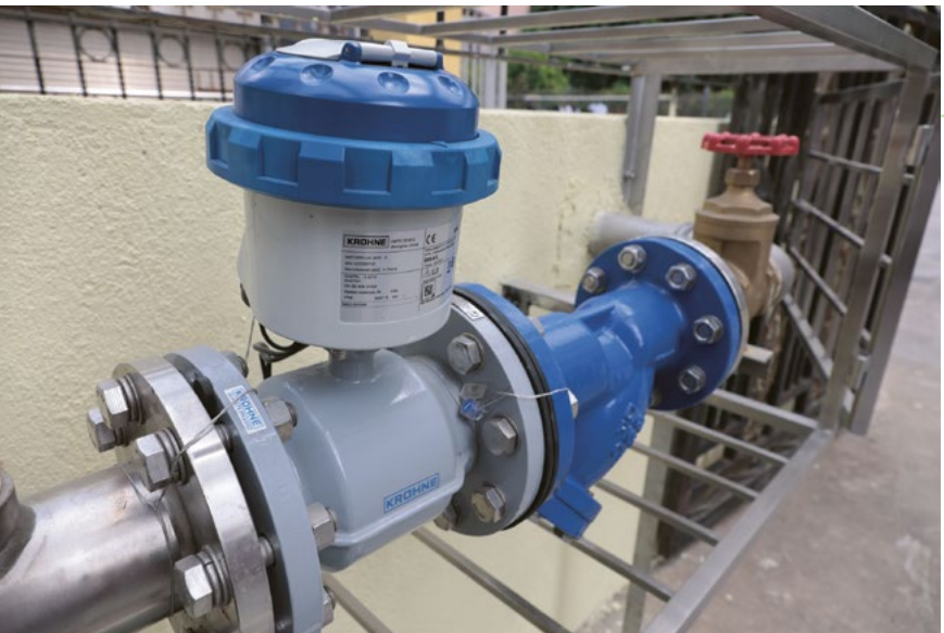
▲ A master meter measures the total amount of water supplied by the WSD in housing estates
