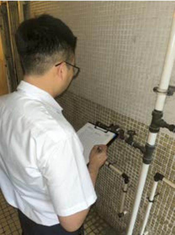
▲ A licensed plumber inspects and records whether the pipe materials and connections outside a building comply with water safety standards.
