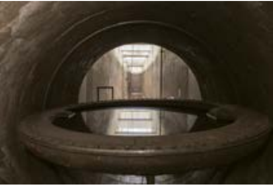
▲ The butterfly valve inside the Dongjiang water main controls the flow of water by a remote switch.
