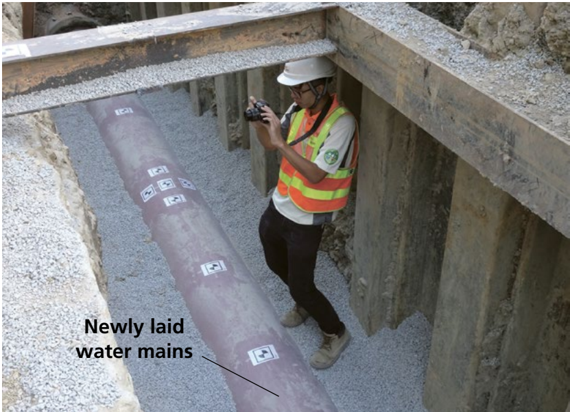
▲ Staff acquiring data by photogrammetry
