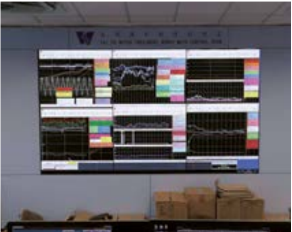
▲ A screen on the wall of the control room displaying the real-time water quality parameters of each process.
