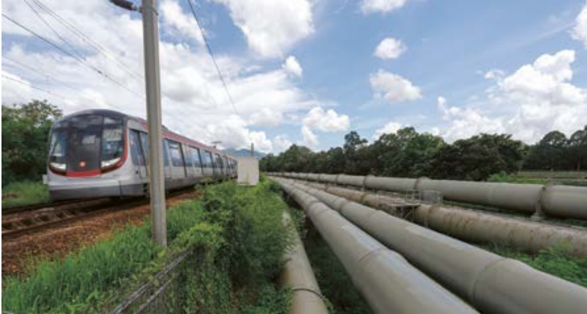
▲ The raw water is transferred from the MWRWPS to downstream water treatment works and impounding reservoirs via pipelines. These pipelines, over two metres in diameter, are of a rarely seen above-ground type.
