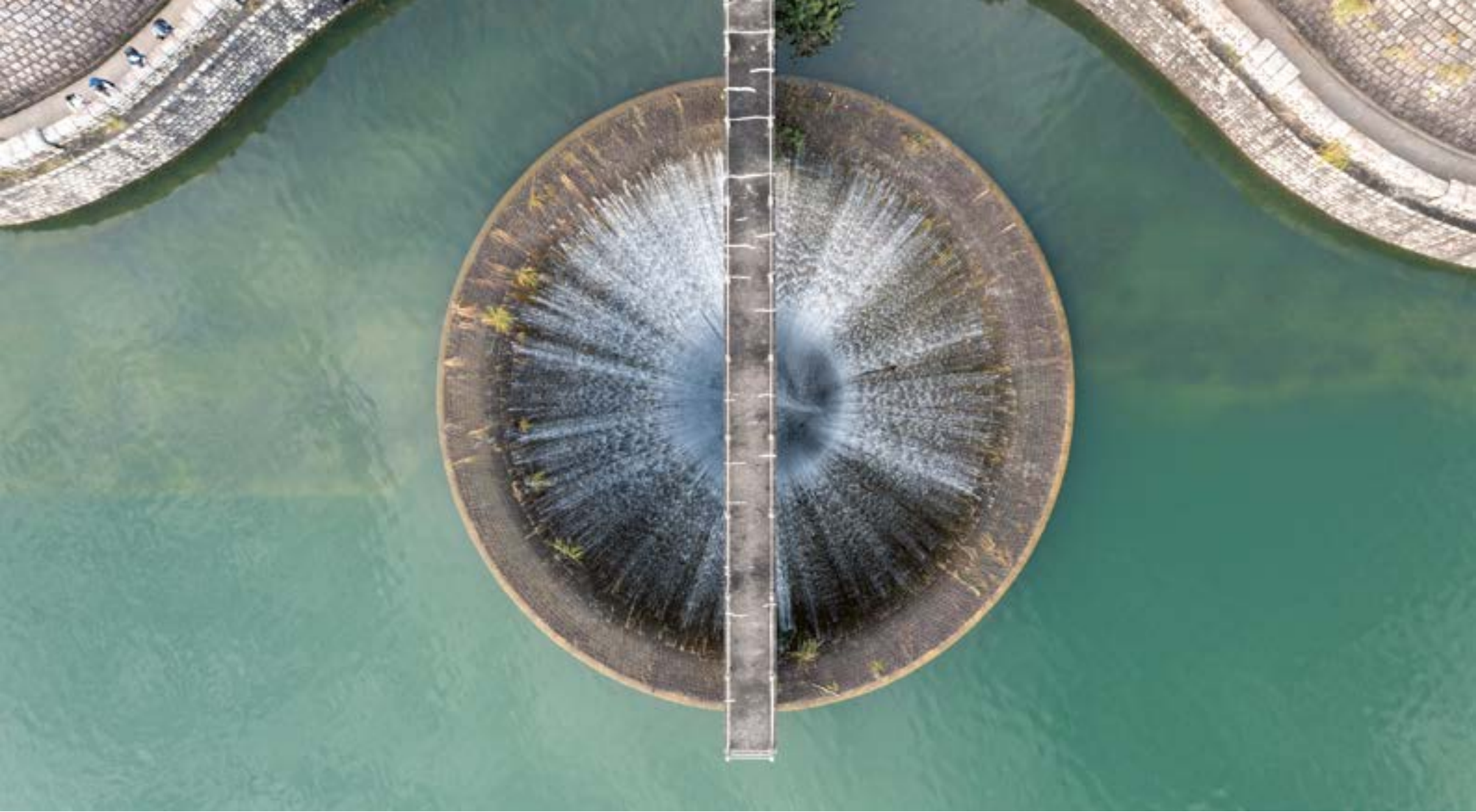
▲ Aerial view of the bellmouth spillway at the Shing Mun Reservoir
