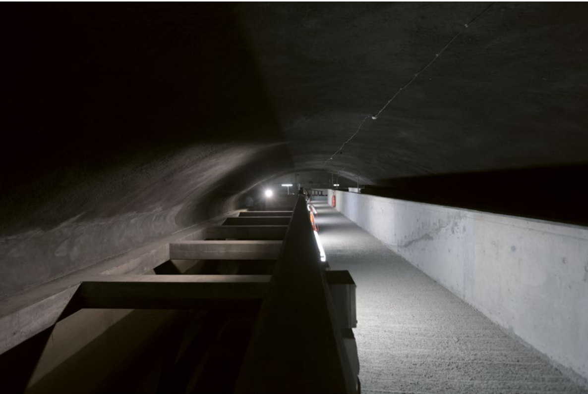
▲ The salt water service reservoir within the cavern was designed in the form of a 100 metre long tunnel
