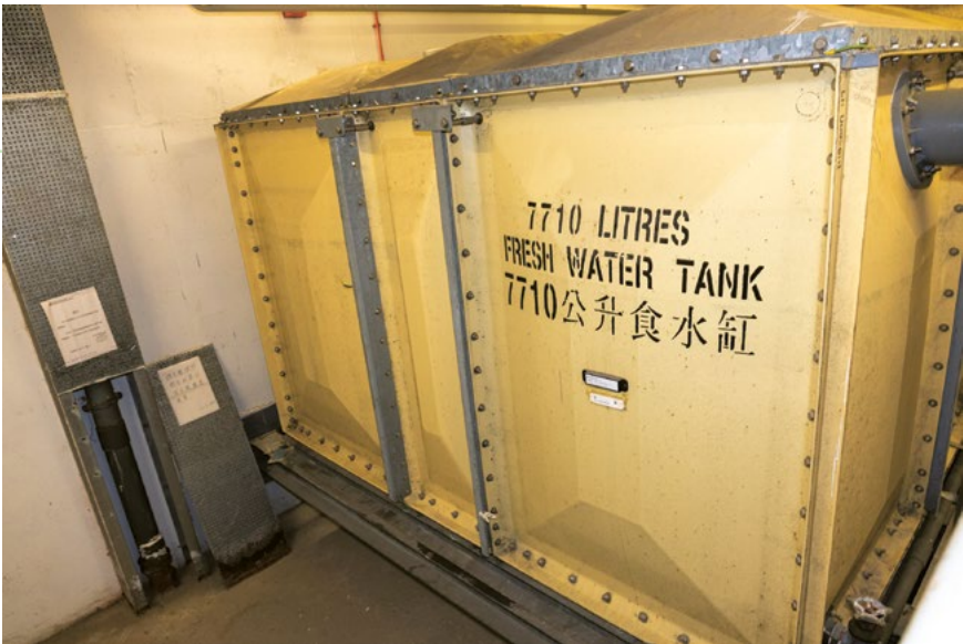
▲ Fresh water storage tanks in buildings
