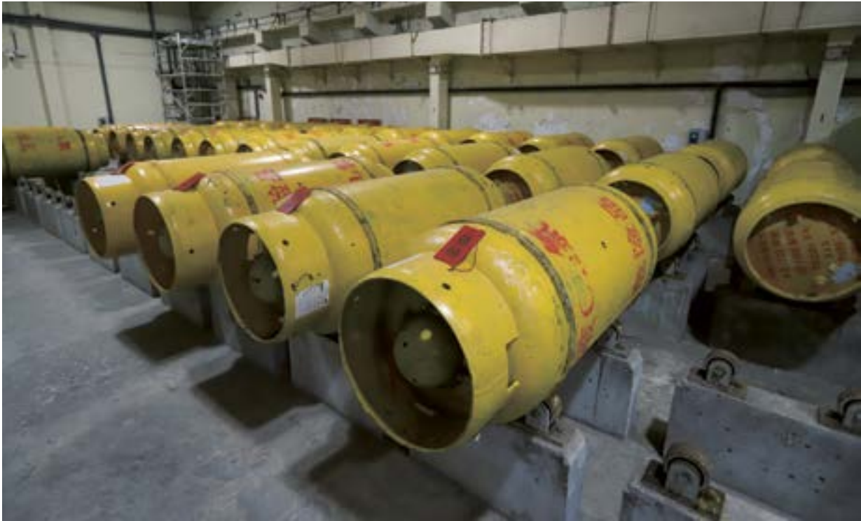
▲ Before on-site chlorine gas generation became available, liquid chlorine was required to be stored at water treatment works.
