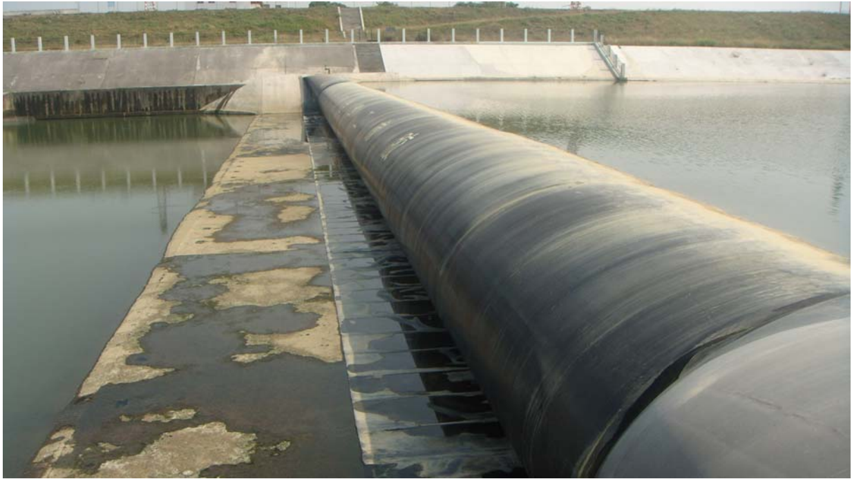
Photo 7 – The rubber dam of Shima River Sewage Diversion Works
