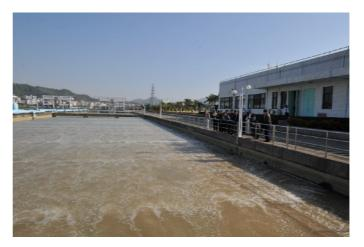
Reservoir. The Bio-nitrification Plant was constructed before the Dedicated Aqueduct project for the purpose of removing the ammonia present in the incoming Dongjiang water. In the Bio-nitrification Plant, the delegation noted that the quality of Dongjiang water received in Shenzhen Reservoir had improved significantly since the commissioning of the Dedicated Aqueduct. Due to the improvement in the water quality, the Bio-nitrification Plant was operated at a lower aeration rate on a need basis
