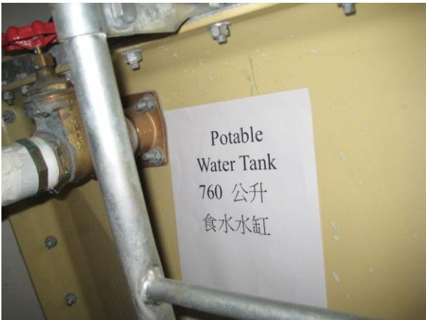
Photo 1. - DN50 inlet pipe
