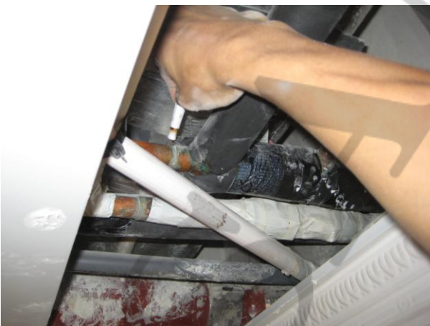
Photo 5- 28mm/Lawton/copper branch tee
