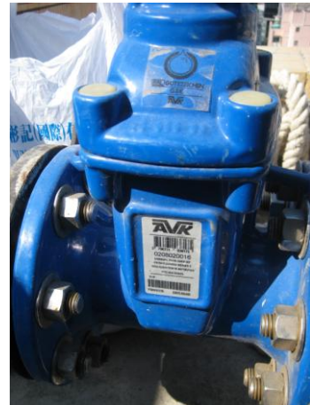
Photo 6 - Gate valve / AVK
