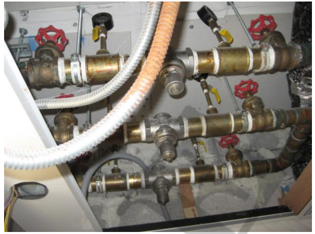
Photo 8 -50mm /PRV/ hot water
