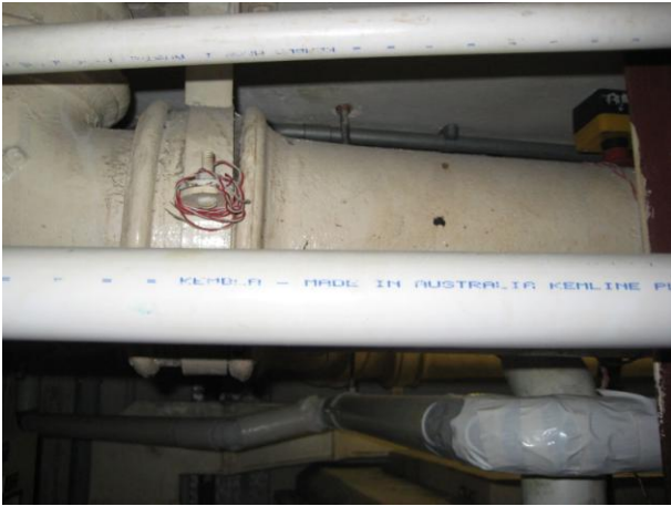
Photo 1. - DN50/Copper/Kembla
