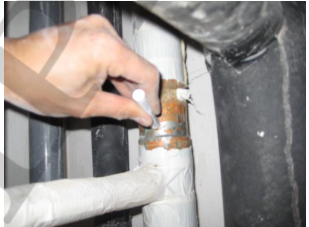
Photo 4. -50mm/Copper branch tee
