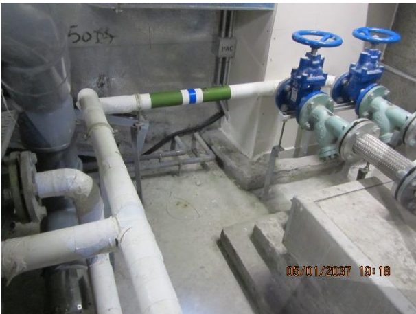
Photo 3. - 67mm/copper branch tee /Lawton
