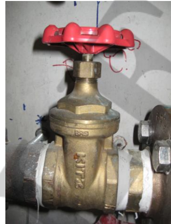
Photo 2. - DN50/bronze gate valve /Kitz
