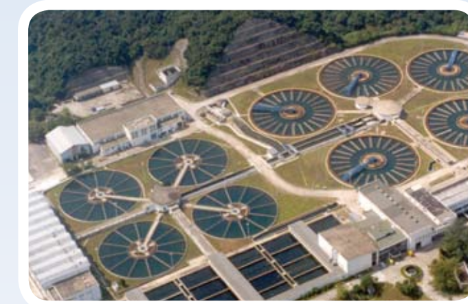
Sha Tin Water Treatment Works
