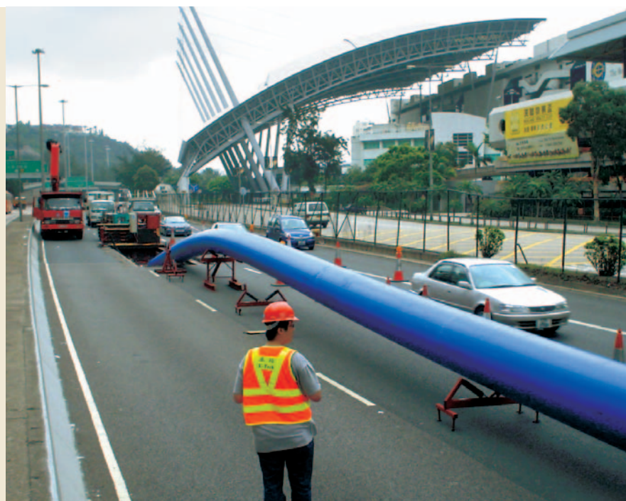
利用無挖坑技術以減少掘路。 Using trenchless technology to minimize road opening work.
