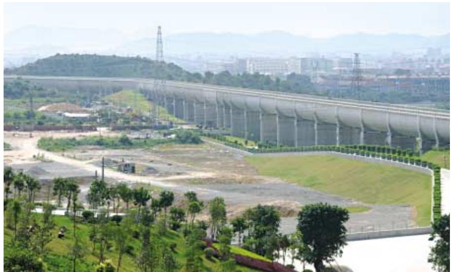
一段密封式輸水管道的外貌。 A section of the closed aqueduct.
