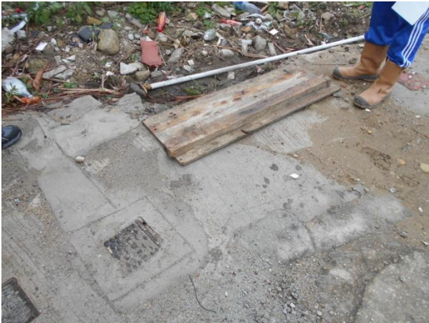
Photo 1 – [Item 1] Position of Connection Point
