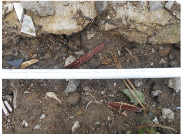
Photo 2 – [Item 2] 25mm KEMBLA copper pipe
