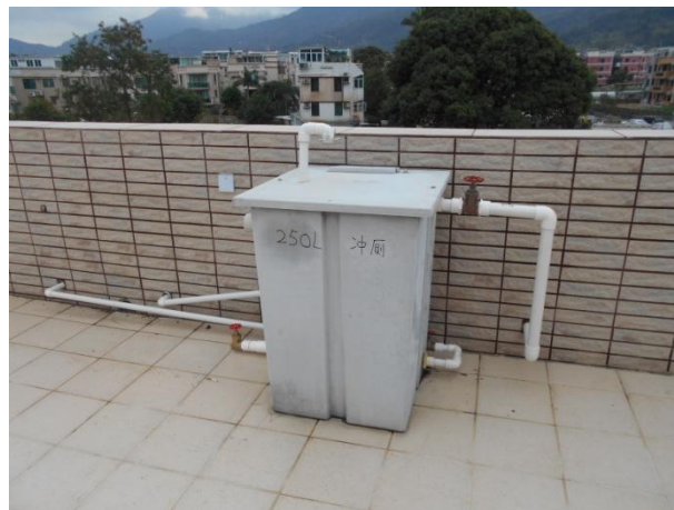
Photo 12 - [Items 21-29] Water Tank
