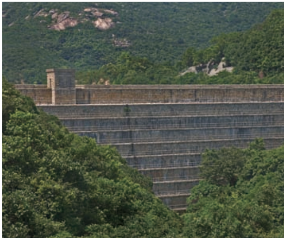
大潭上水塘水壩 Tai Tam Upper Reservoir Dam 1883-1888
